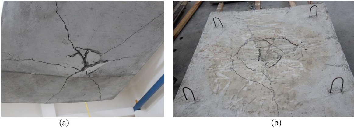
Figure 11. Crack patterns of panel J50 (a) flexural crack (b) tangential crack
