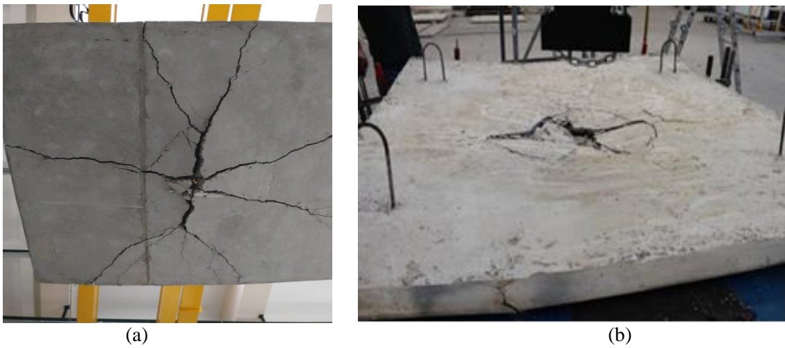
Figure 12. Crack patterns of panel J70 (a) flexural crack (b) tangential crack
